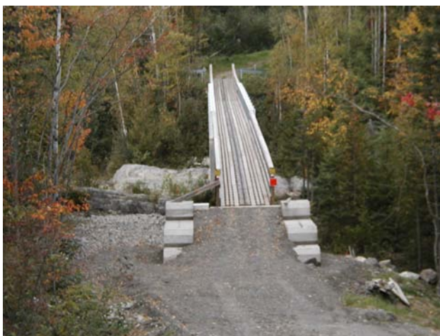
New ATV/Snowmobile Bridge over the Moose River in Rockwood (BP&L Photo)
